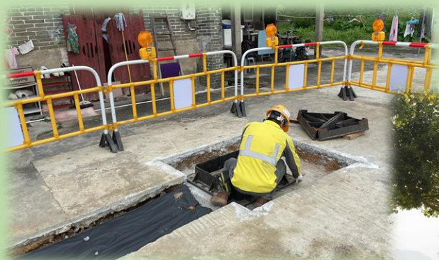
塘肚村污水渠鋪設工程 Sewers Laying at Tong To Village
