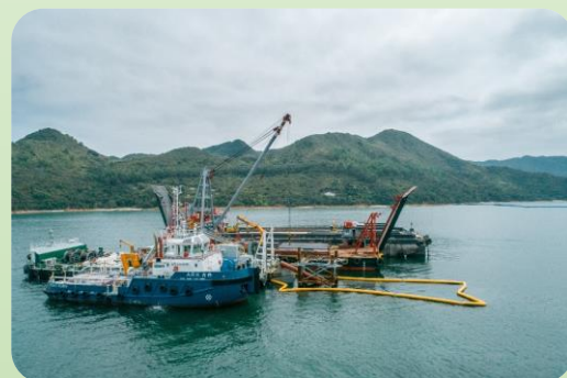
建造海底排放管 Construction of Submarine Outfall
