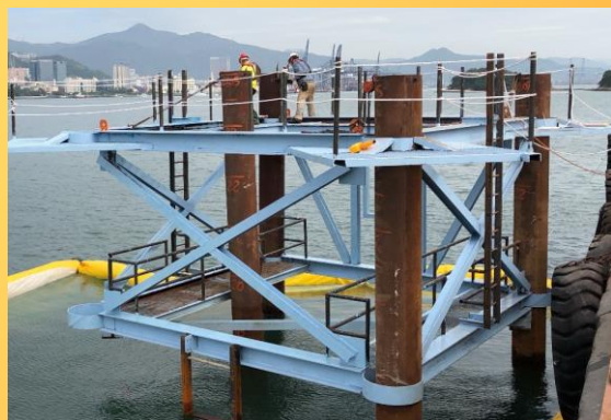
建造海上臨時工作台 Construction of Temporary Working Platform at Sea
