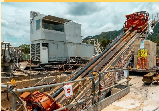
建造海底排放管 Construction of Submarine Outfall
