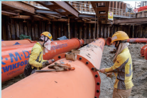
新污水處理廠組件場外組裝 Off-site Fabrication of Components for New Sewage Treatment Works
